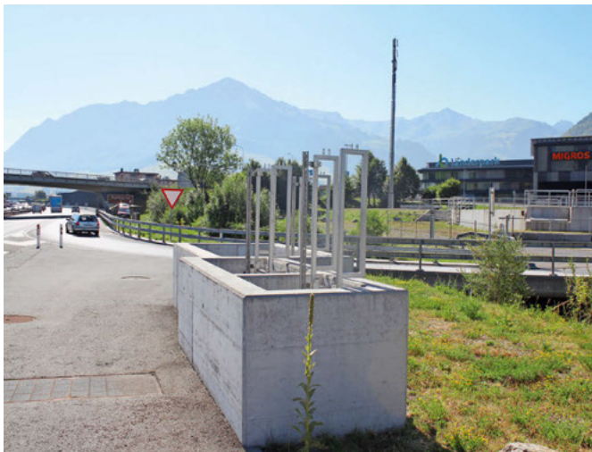
4 | SABA Spichermatt [Sauber+Gisin Engineering AG, 2017]. 4 | SETEC de Spichermatt [Sauber+Gisin Engineering AG, 2017].
